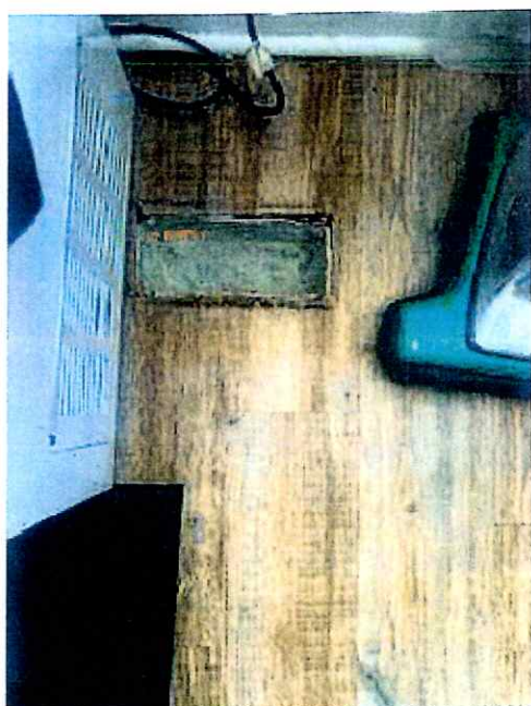
Duct Sealing view from above
