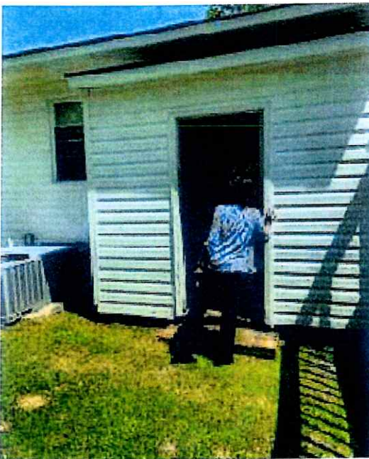
Staff member is observing the Hot Water Heater and Insulation.
