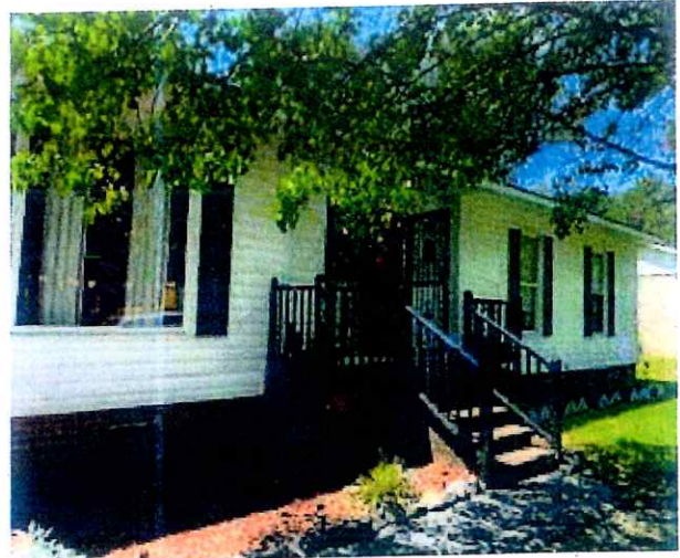
Blower Door View from Outside of Client's Weatherized Home.
